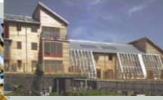
1999 - 2001 INTEGER project, UK Five demonstration social housing schemes using low carbon building and energy technologies
